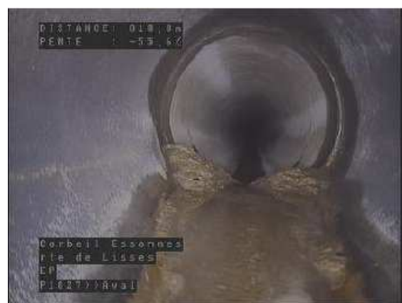
Route de Lisses - Infiltration importante
