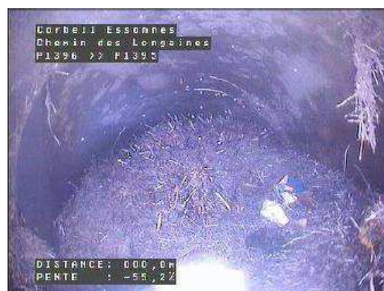
Chemin des Longaines - Obstruction
